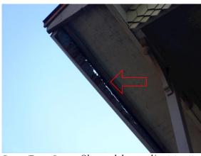
Gutters/Down Spouts: Observed damaged/rustet gutters
