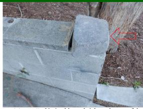
Retaining Walls: Noticed loose brick on the top of the retaining wall
