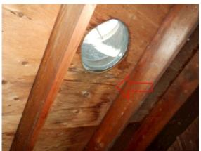
Attic Framing/Sheathing: Water staining on roof sheathing, mainly around vent penetration
