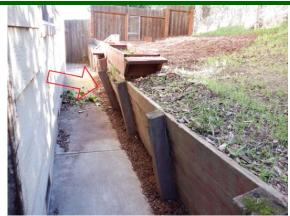
Retaining Walls: The retaining wall was showing signs of bowing/leaning
